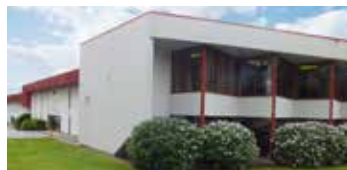
BURNABY LAKE INDUSTRIAL CENTRE, BURNABY
